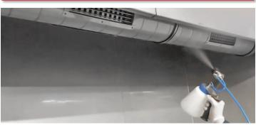
**Ventilation systems:** For the targeted disinfection of the air inlet you will find the nozzle for the larger throw range in the scope of delivery.
